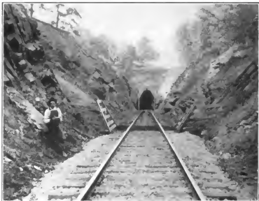
TWIN TUNNEL BETWEEN BELLTON AND PENROD On Louisville & Nashville Railroad
